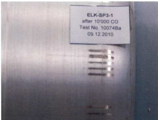
Photo 4: Moving contact side of main contact
